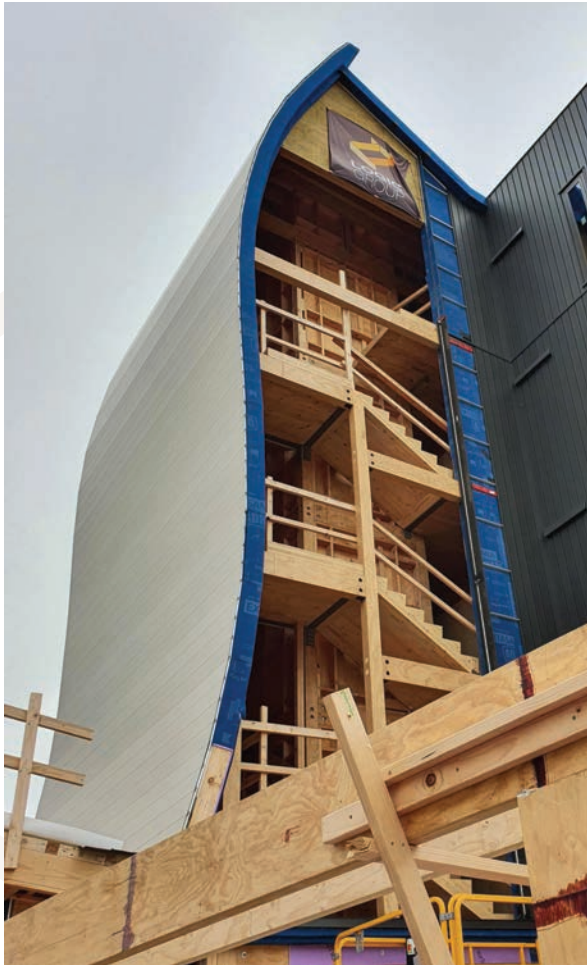
Construction as of 3 November 2021
