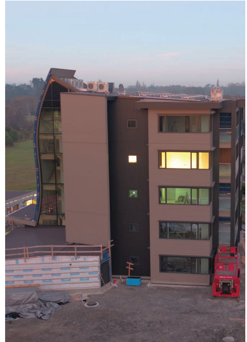
Construction as of 03 May 2022
