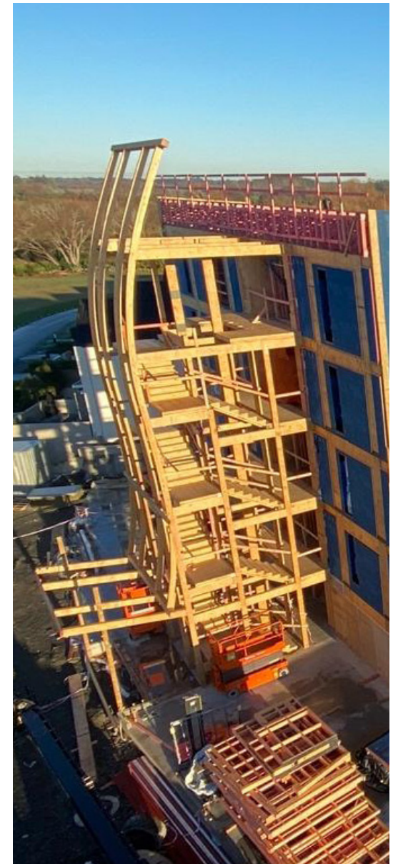
Fig. 21 - Curved Glulam Column Being Installed
