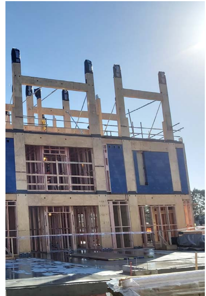
Fig. 26 - Photo showing first two levels of H frames
