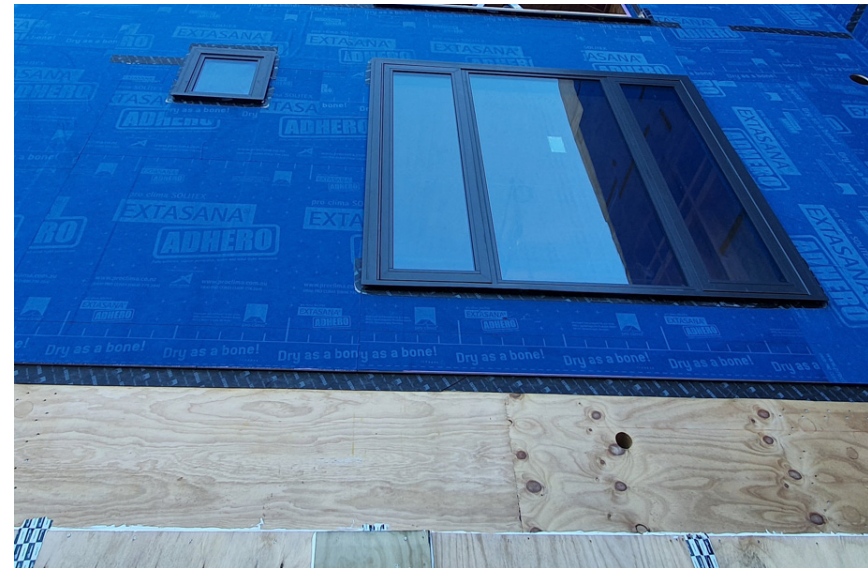
Fig.5 - Wall membrane applied over the Rigid Air Barrier – Clearwater project
