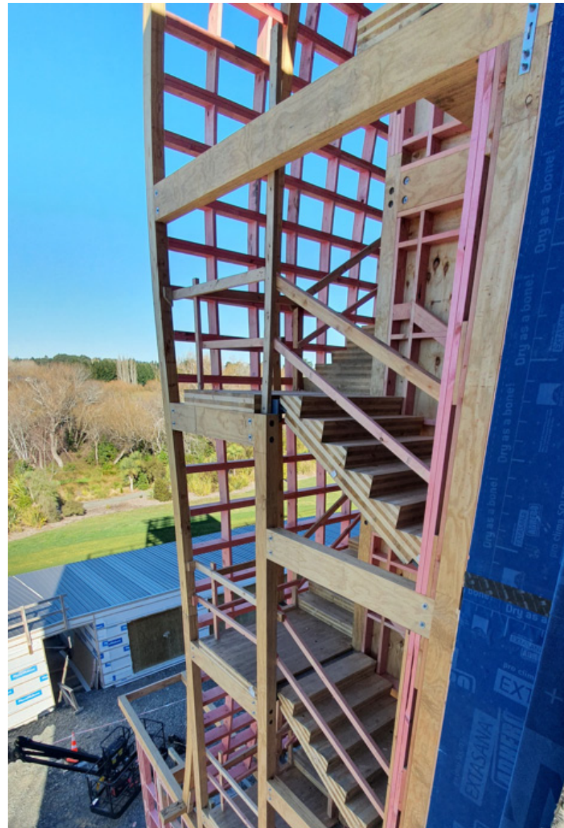
Fig. 10 - Curved wall to curtain wall interface
