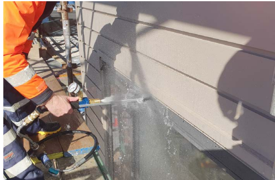
Fig. 9- AAMA 501.2 Site Hose Testing – Clearwater Quays
