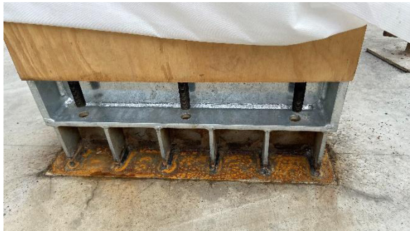
Fig. 30 - Photo showing portal column base connection on site
