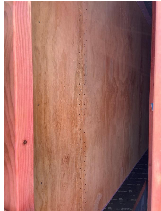
Fig. 33 - Photo showing plywood sheet edge nailing
