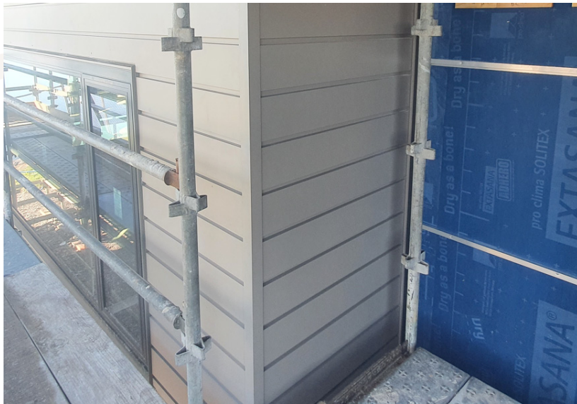
Fig.4 - West Elevation External Cladding Site progress – Clearwater project
