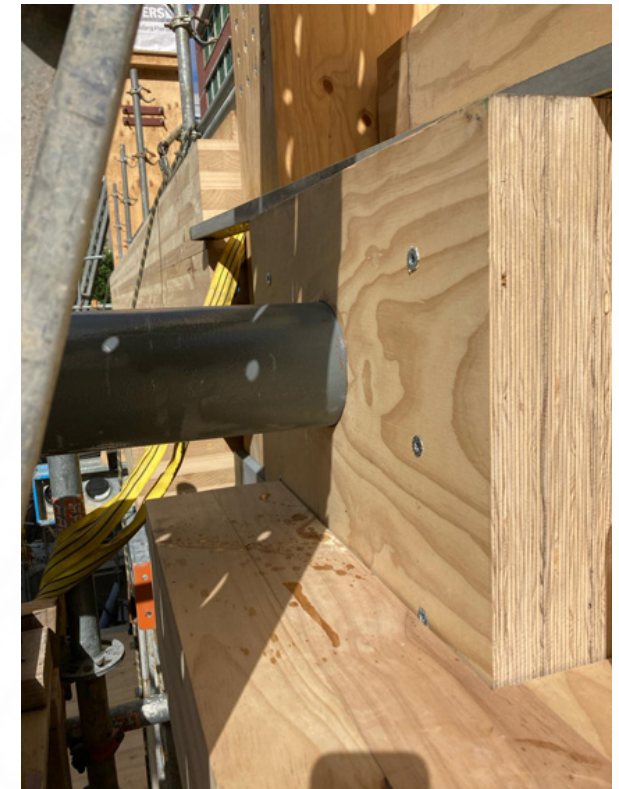
Figure 3: 150 diameter steel pin installation
