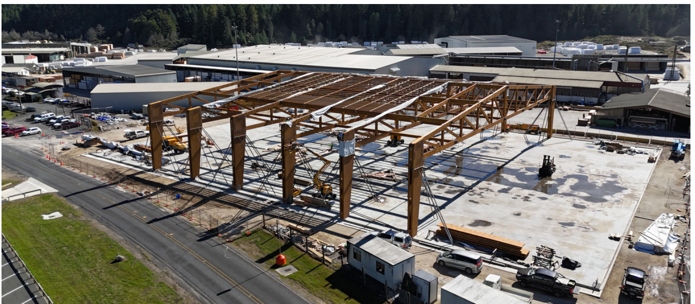
RST Dry Store - Build in progress
